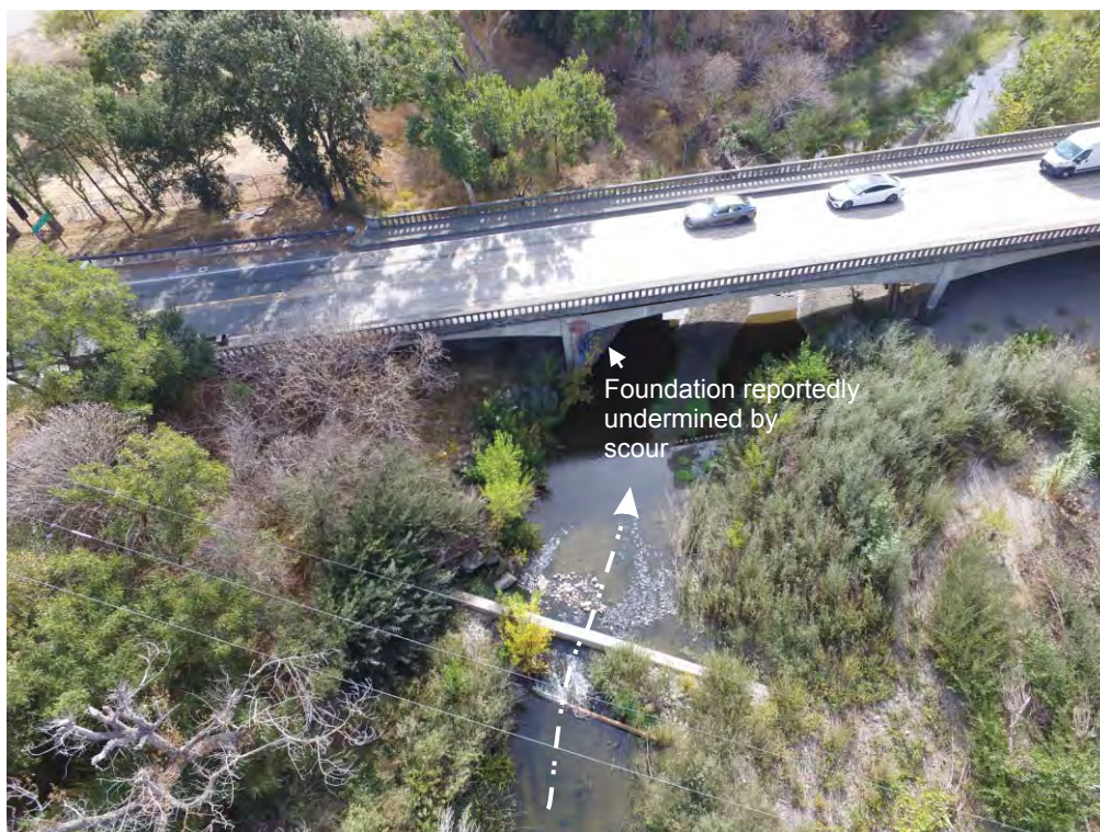
Aerial Drone Image 2. Southerly view of 1939 Highway 84 bridge across Arroyo de la Laguna near southeast corner of campus approximately 1000 feet downstream from overtopped bank location. Note concrete weir to moderate flow. Flow was reportedly blocked by vegetal debris causing flood water to nearly overtop the deck.
