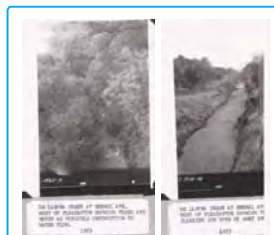
Dramatic example of channel modification that occurred on Arroyo De La Laguna at Bernia Avenue in 1953. The photo on the left shows the reach before riparian vegetation clearing, while the photo on the right shows the same reach after clearing by the Army Corps of Engineers (Source: Alameda County Resource Conservation District).
